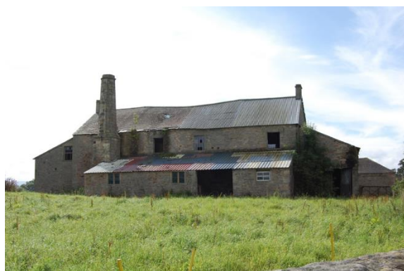
Moss House Mill
